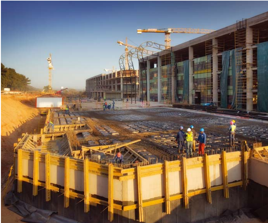
■ Work is underway on the R1,3 billion head office complex for the Department of Foreign Affairs in Pretoria. The R1,3 billion structure topped out in August and Concor is scheduled to complete the project in May 2009
