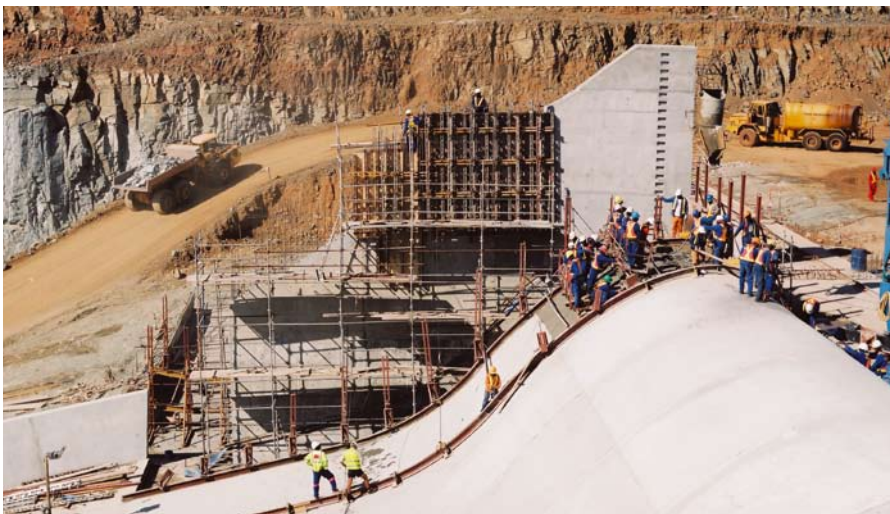
■ Concor, in joint venture with Group 5 and Swaziland-based Inyatsi Construction, has successfully completed the upstream components of the LUSIP Dam Project in Swaziland
